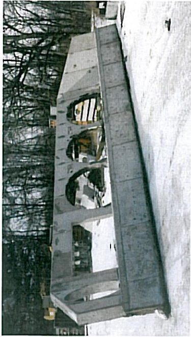
Special Headwall with 4- 48" pipe openings and 1- box culvert opening
