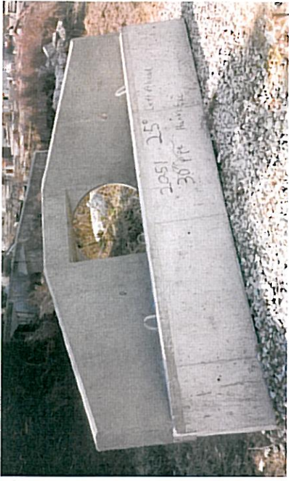
30" Pipe Headwall Flared with 25 degree angle
