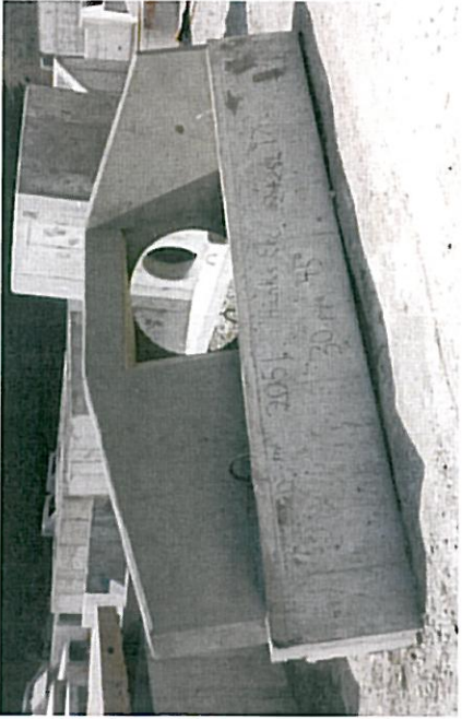
30" Pipe Headwall Flared with 45 degree angle
